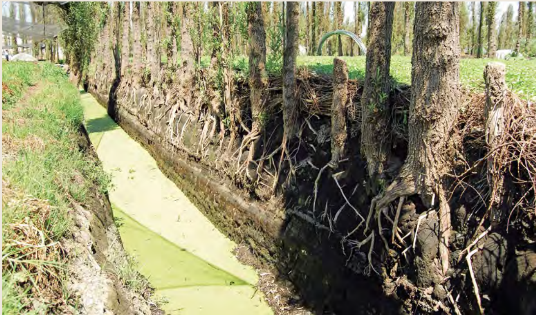
FIGURE 10. The roots of the ahuejotes interlock preventing the banks, tall and nearly vertical, as in this case, from disintegration. Their tops are almost always covered with grass, which is normally of spontaneous growth.
