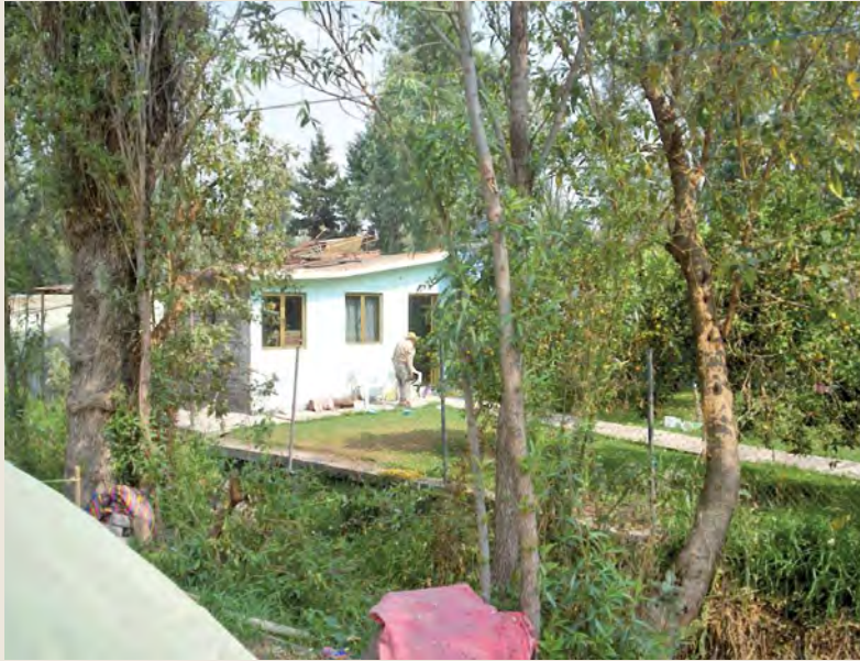
FIGURE 72. Formal house, with all services, good finishes and domestic garden in one of the chinampas in the south of sector 9, next to the Canal Nacional.
