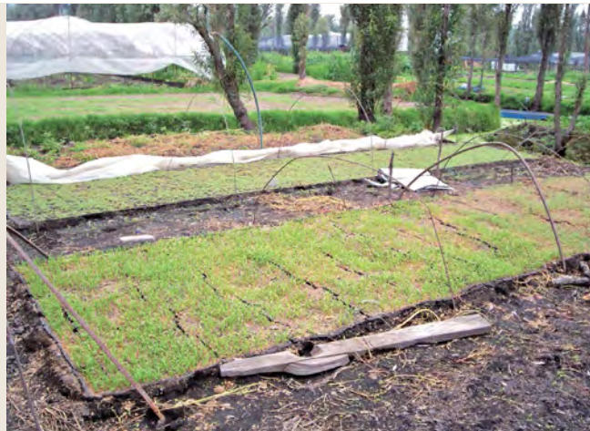
FIGURE 74. Construction of micro-tunnels over almácigos . The plastic is supported on several curved steel rods as can be seen to the right of the photo.
